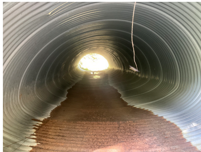
Looking Downstream Through CMP
